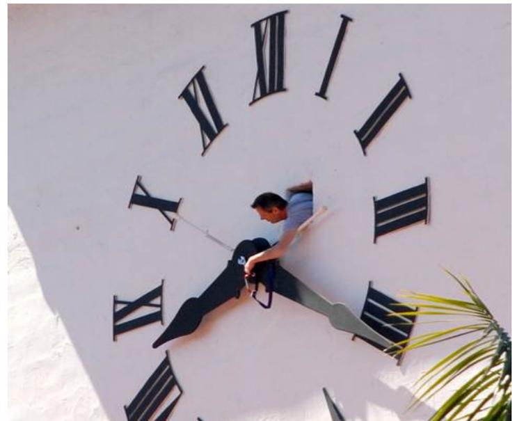
Mostyn is not standing on the floor but is perched on a ledge that runs along the inner wall. (I tied a bungy cord to his ankles, in the event something happened we could retrieve him on the rebound.) The wrench and minute hand were secured to nylon straps to prevent them from falling to the ground. Working from both sides of the dial, the nut was removed in a surprisingly short time.
